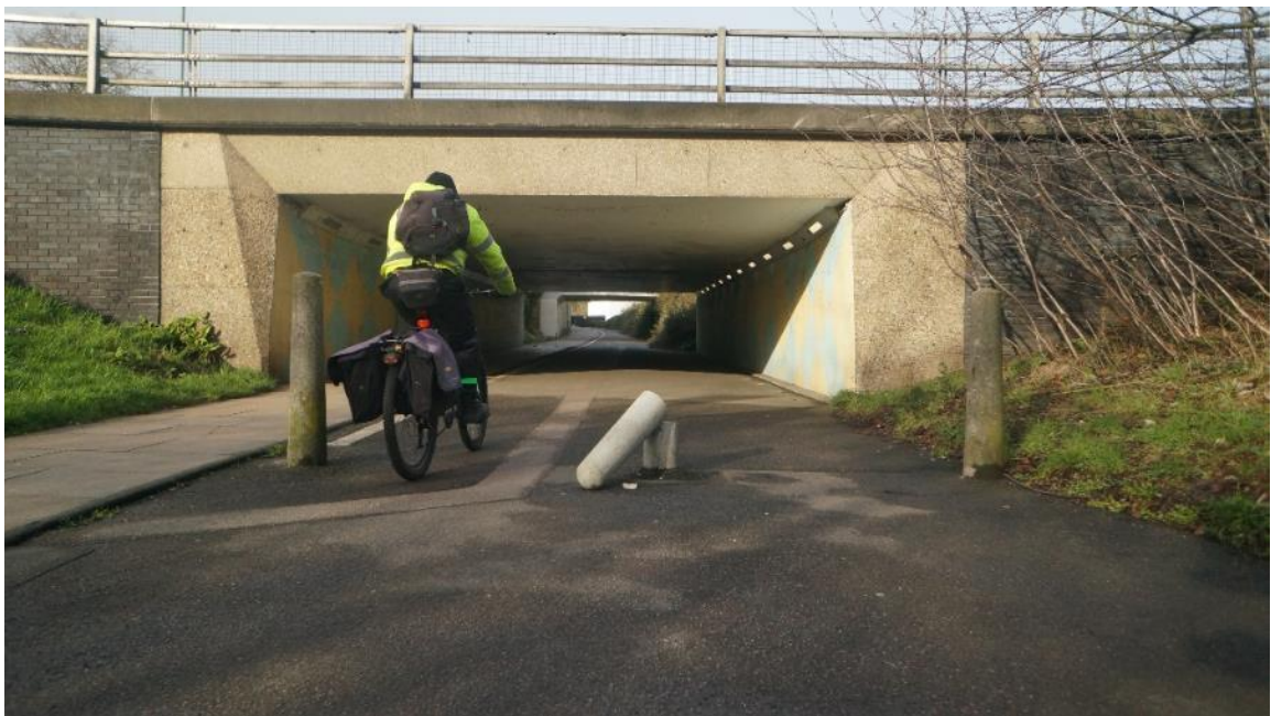
Figure 3-3: Example of a grade-separated junction underneath Fifth Avenue
