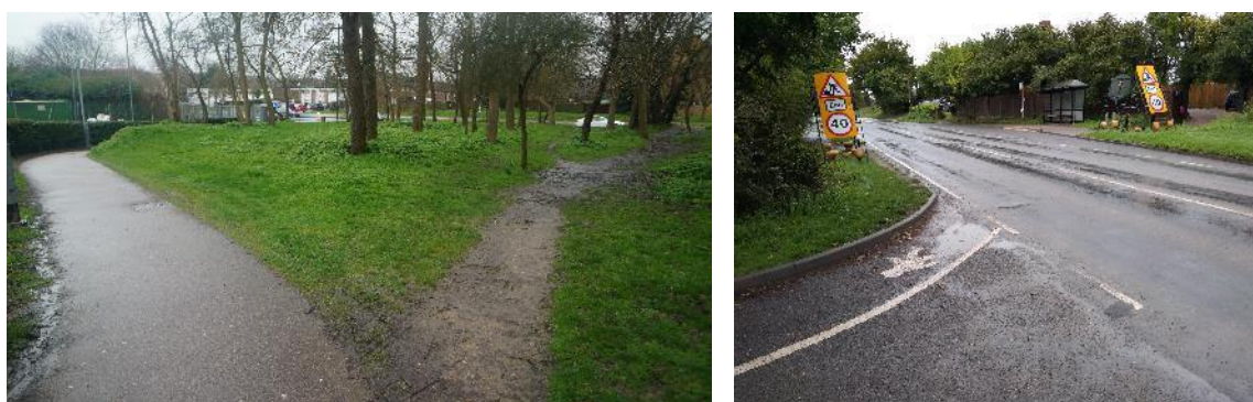
Figure 7-7: Pedestrian Desire Line towards Velizy Avenue (left), and sub-standard footway provision in Templefields
